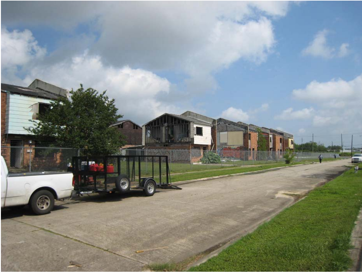
4/29/16 Abandoned and blighted homes
