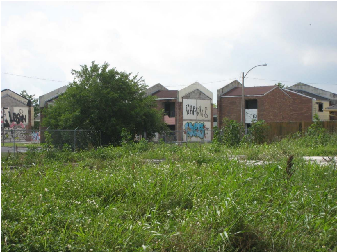
4/29/16 Abandoned and blighted homes
