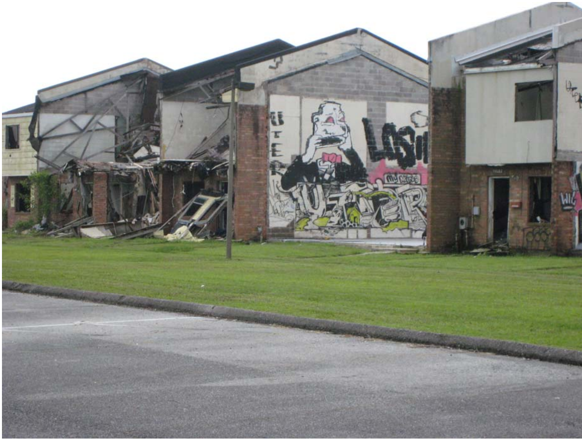
4/29/16 Abandoned and blighted homes
