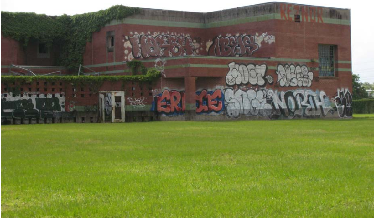
4/29/16 Abandoned and blighted school building
