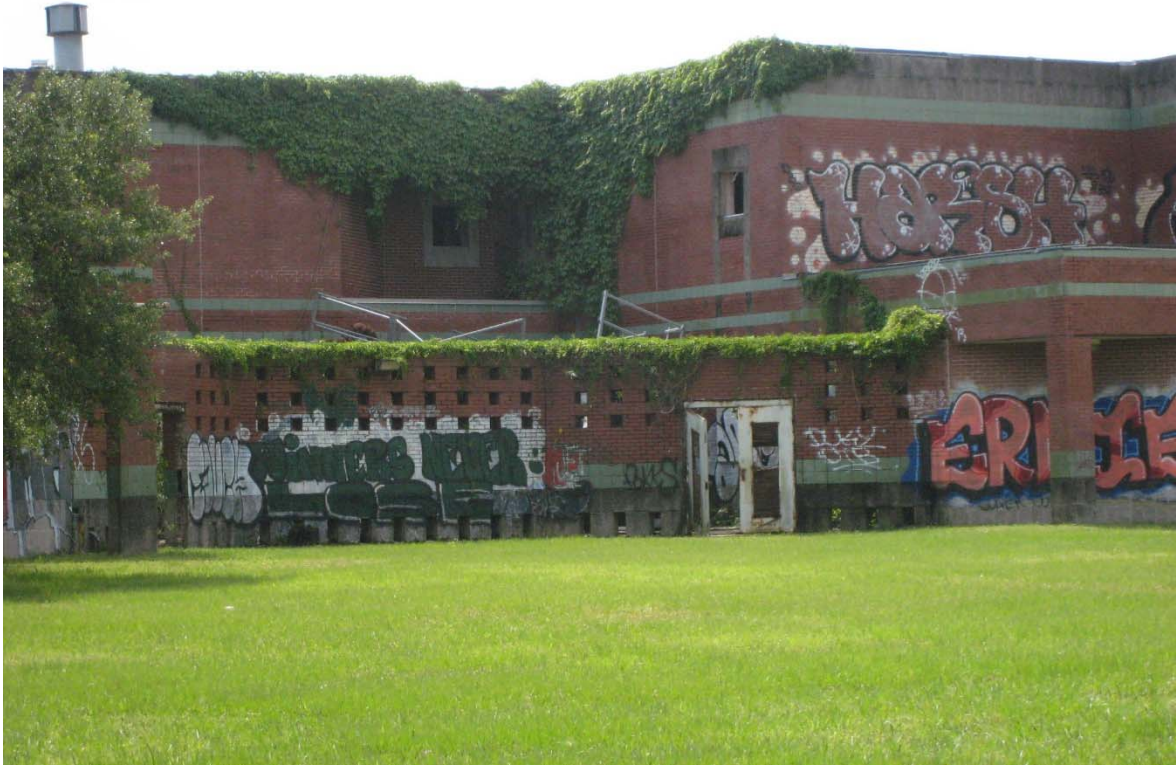
4/29/16 Abandoned and blighted school building
