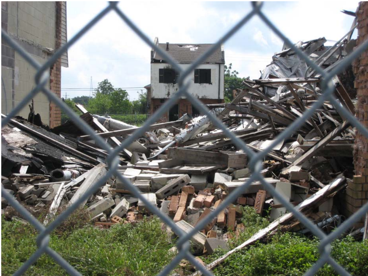
4/29/16 Abandoned and blighted homes
