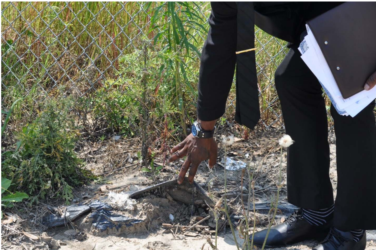
5/10/16 Exposed geotextile mat (indicating the interface between fill and contaminated soil)
